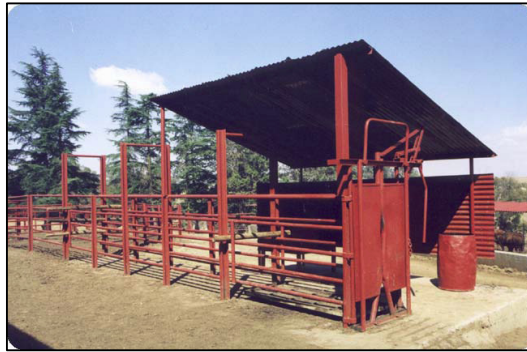
Figure 2.2 Typical working area (after Breedt, 2003)
